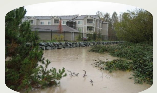
Properties built above the base flood elevation are protected from most flooding events.
